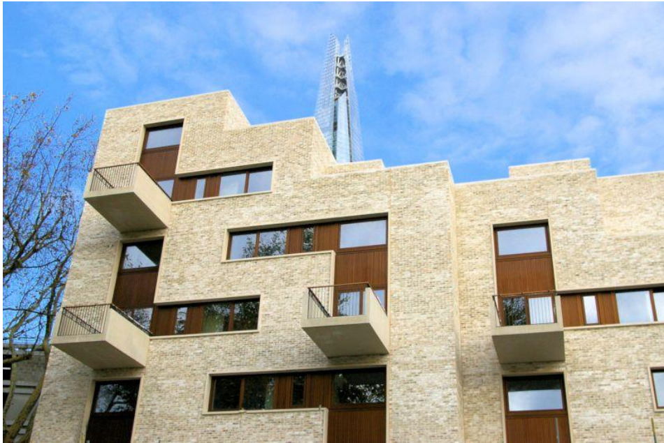
The south elevation of Weston Street. Image: Schöck Ltd, royalty free.
