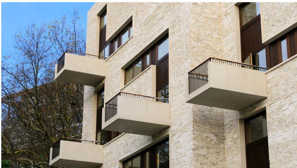
Large and heavy cantilevered concrete balconies. Image: Schöck Ltd, royalty free.
