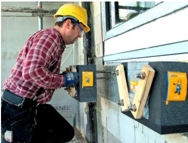
[Isokorb type R installation.jpg]
