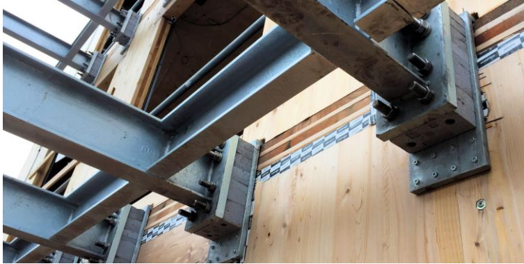
KST modules and CLT in position – Courtesy of KLH UK Ltd
