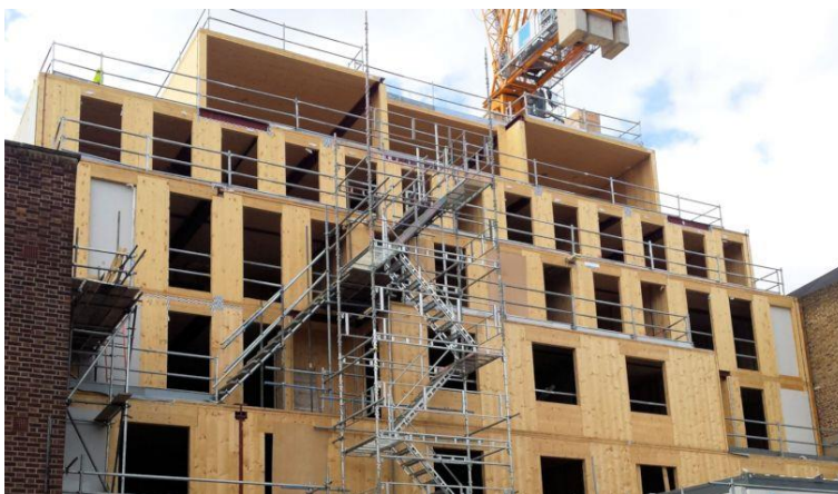
Work in progress at Pitfield Street – Image: Schöck Ltd
