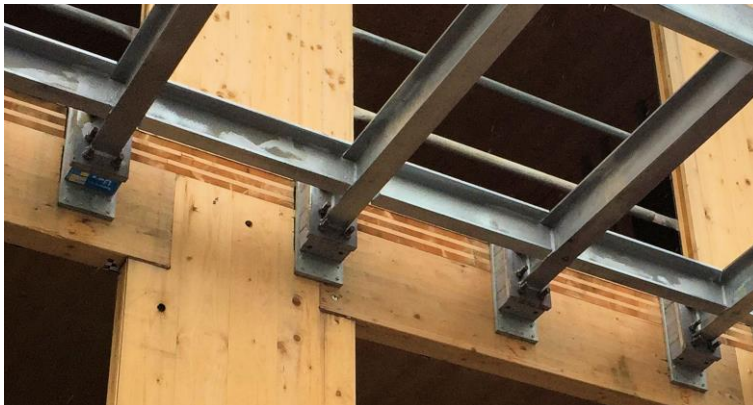
KST modules and CLT in position – Courtesy of KLH UK Ltd
