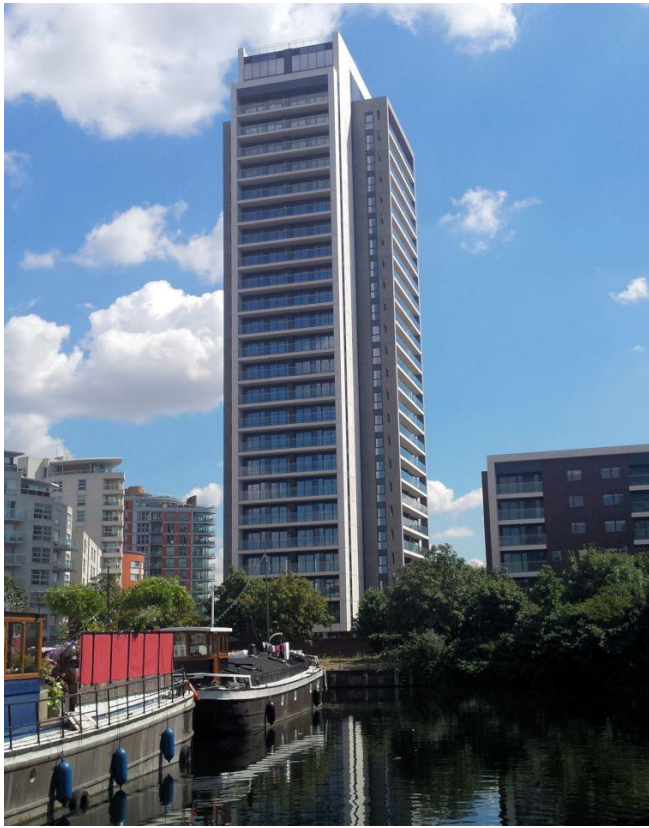
Horizons sits alongside Poplar Dock Marina. Image: Schöck Ltd.
