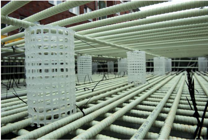
Spacers ensure stability of the multi-layer reinforcement Image: Schöck Ltd.
