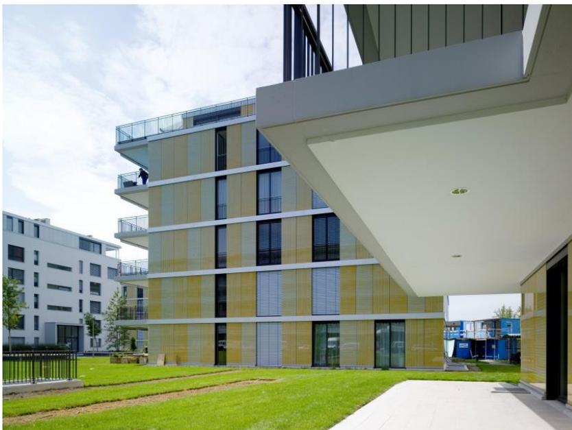
*The Isokorb XT makes it possible for cantilever balcony construction to be built to passive house standards*
