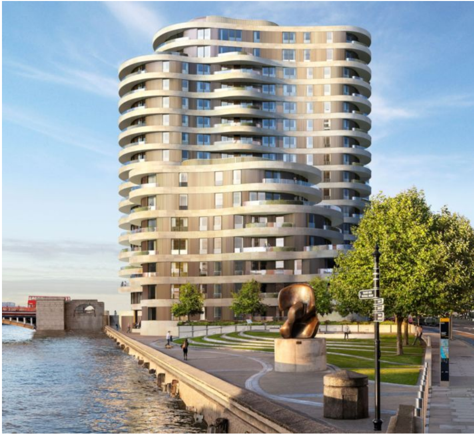
Riverwalk features two organically shaped buildings of 7 and 17 storeys
